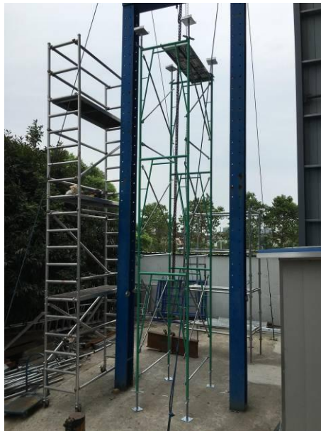
Frame scaffolding assembly
